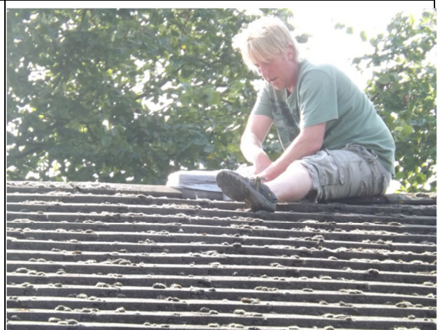
Temporary sealing of ridge vent to facilitate co-pressure testing
