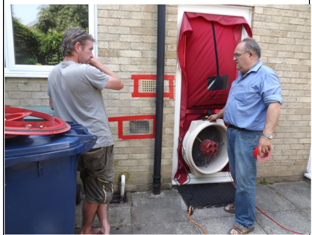
Second fan being installed in entrance doorway of neighbouring property to carry out co-pressure testing
