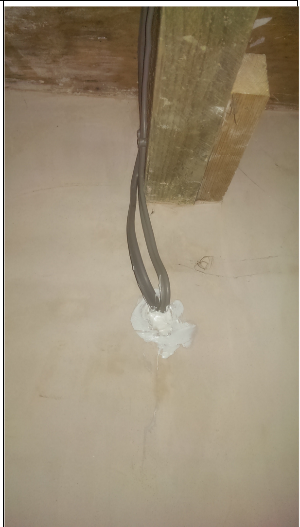
P9) Mastic seal around cable through wall to unheated outbuildings
